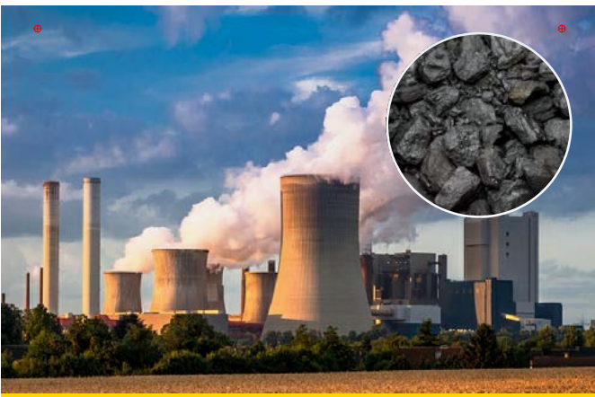
Coal-Fired Power Plant - CO3301-5L02
